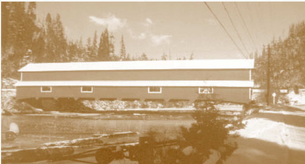
The office bridge at Westfir. Longest covered bridge in Oregon.
