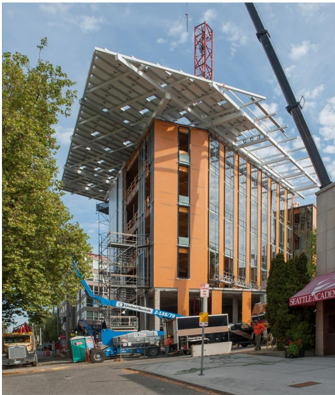
2012-9.8_0009 Bullitt Center Under Construction photo: John Stamets Figure 10—Bullitt Center
