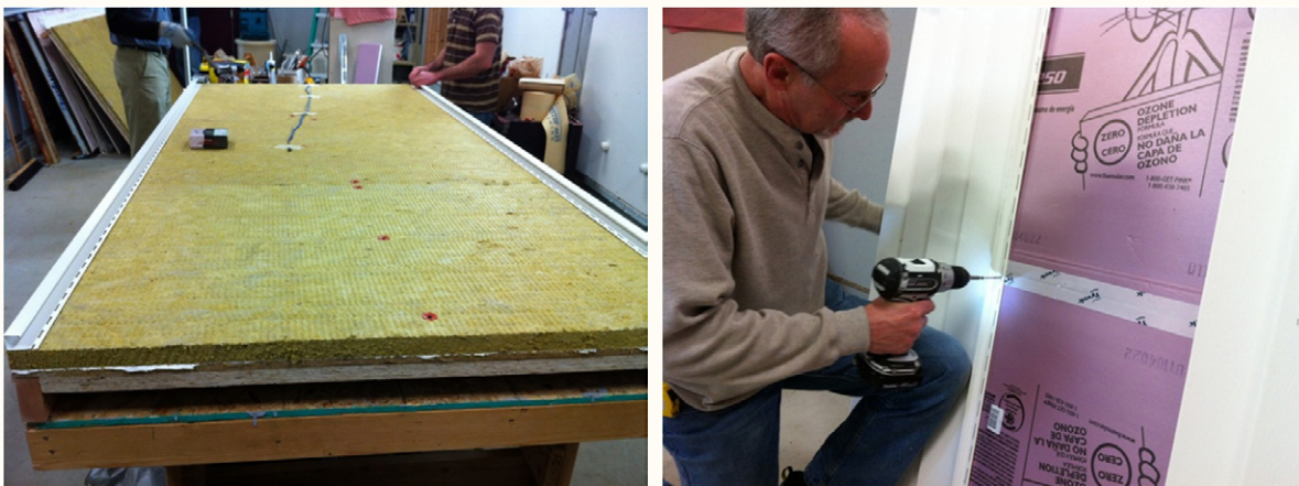
TEST WALLS WITH 1-1/4-INCH MWI (Left) AND 1-INCH XPS (Right)
