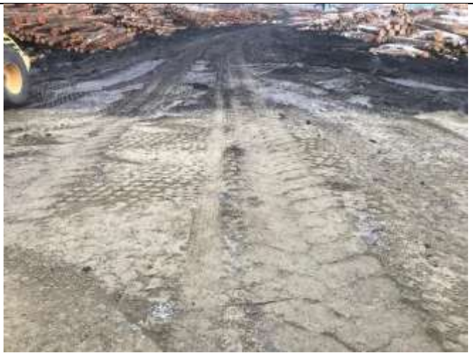
Completed Section vs Previous Logyard
