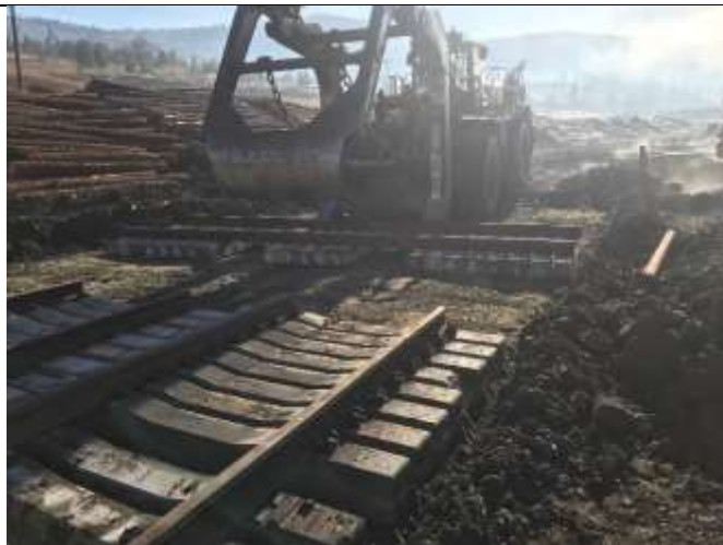
Loader Placing Rail Tie Sections
