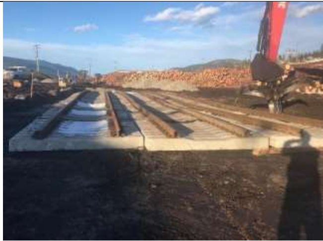
Concrete Rail Tie Sections
