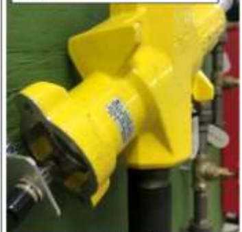
Photo of the valve modification. When the valve is closed it threads through the plywood making the limit switch located on the back.
