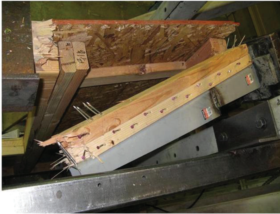
DOUBLE TOP PLATE FAILURE FOR WALL 4A, USING “SHORT” LOAD HEAD)
