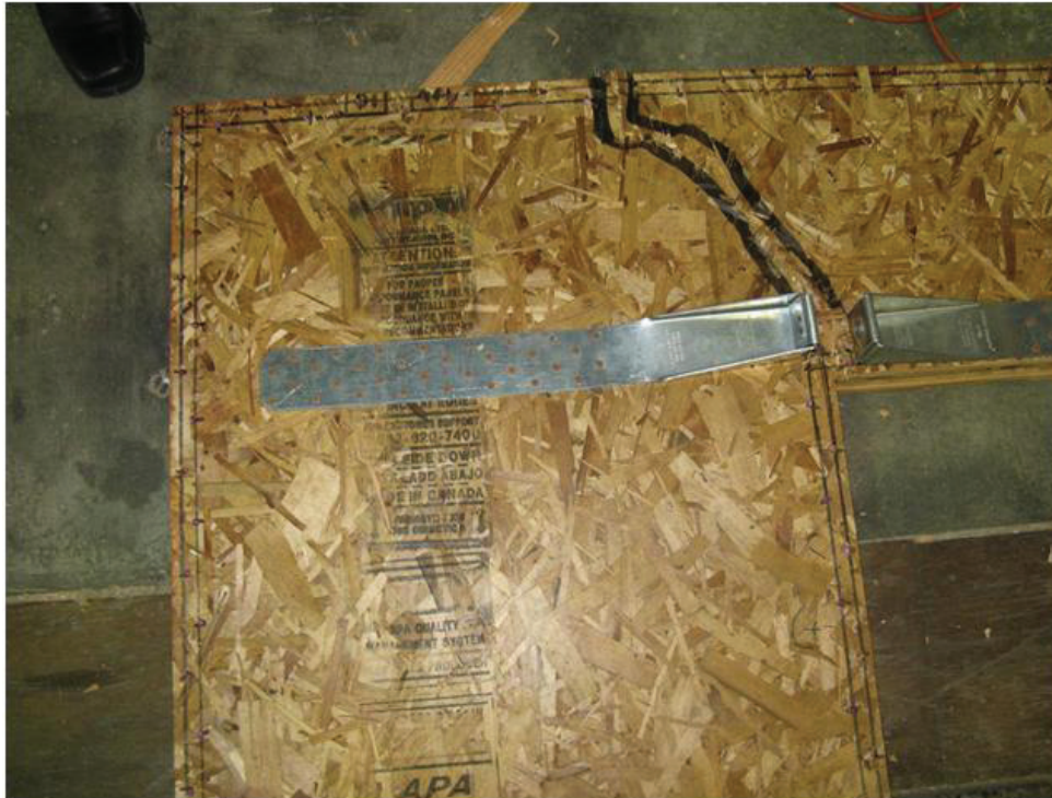
WALL 6A, SHEATHING TEARING, TOP EAST STRAP
