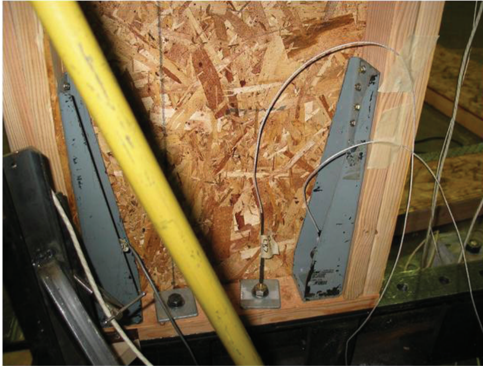
WALL 10B, SHOWING INSTRUMENTED HOLD DOWNS AND ANCHOR BOLTS
