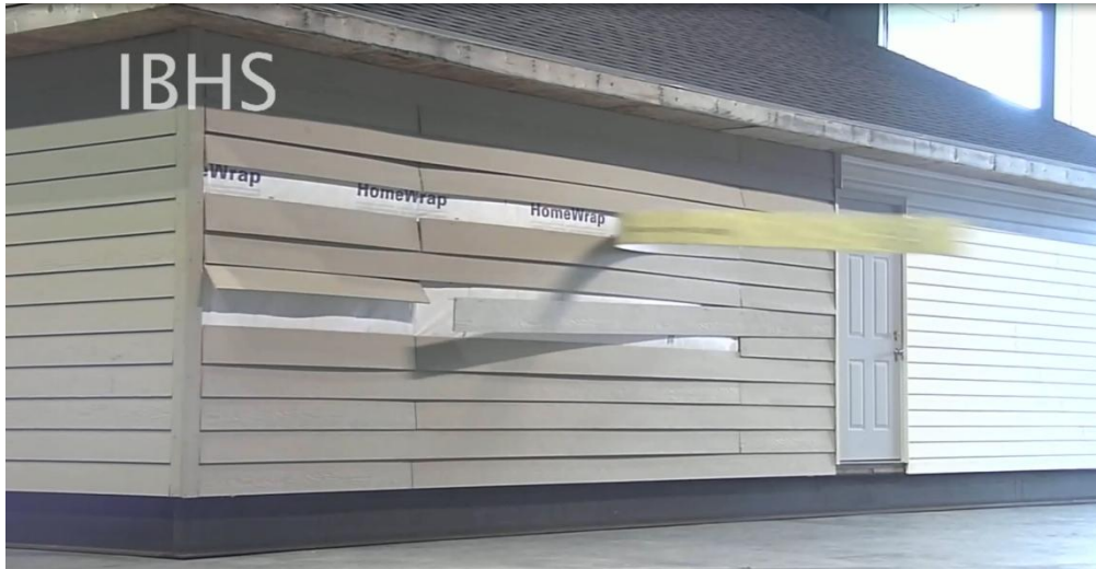
Figure 7. Wall 5 failure during testing at 20° with target gust speed of 48 m/s (108 mph)
