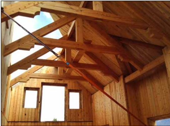
Figure 2. Building being constructed using ICLT panels. Photo by Ryan Smith
