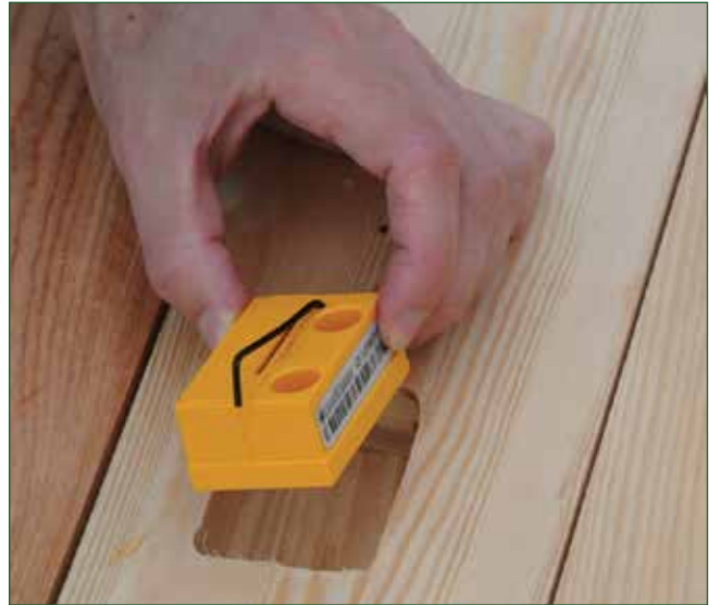
Wireless moisture-temperature sensor being installed in a CLT panel.
