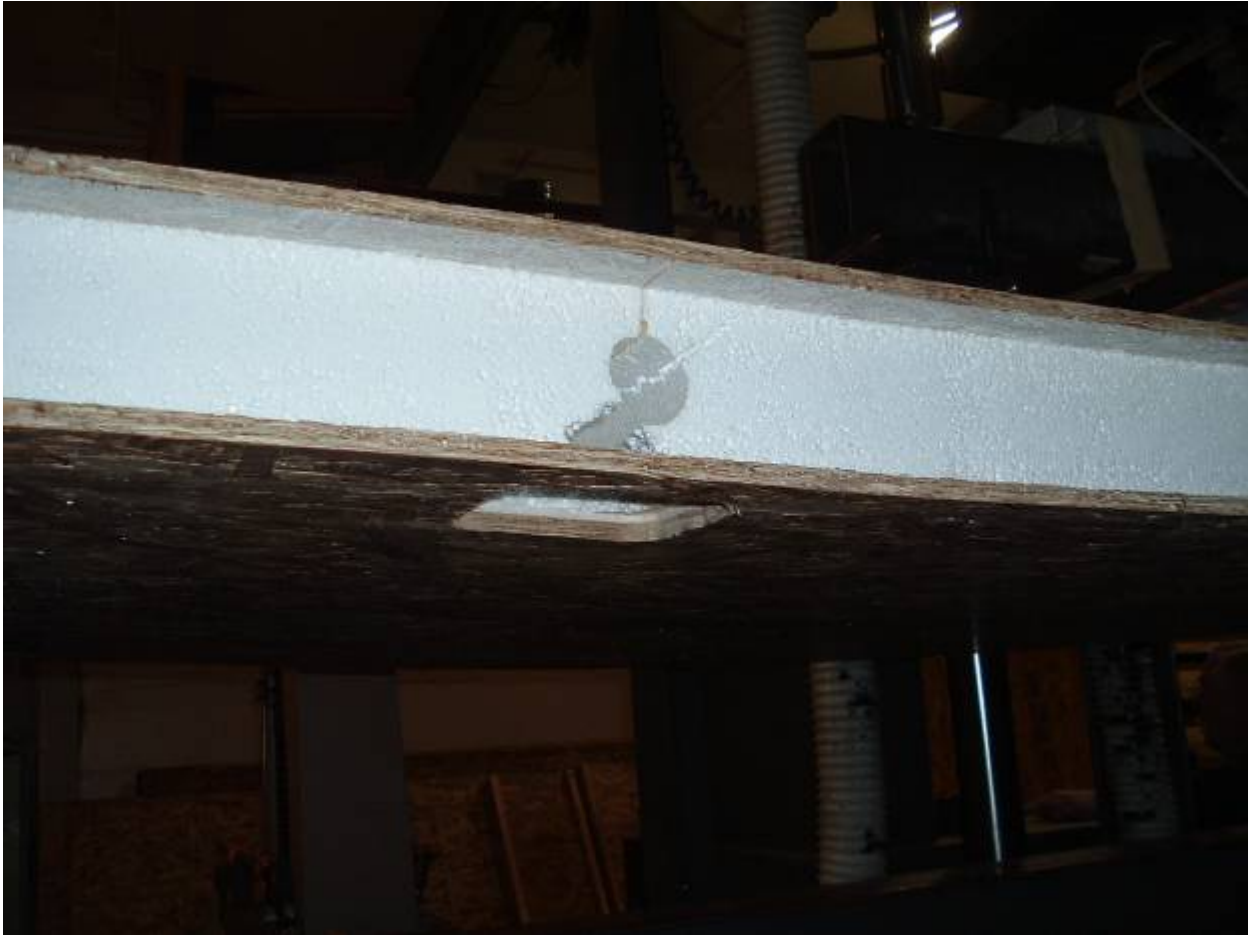
FIGURE C4. TRANSVERSE LOAD TEST (Initial failure on tension side at electrical chase holes - typical)
