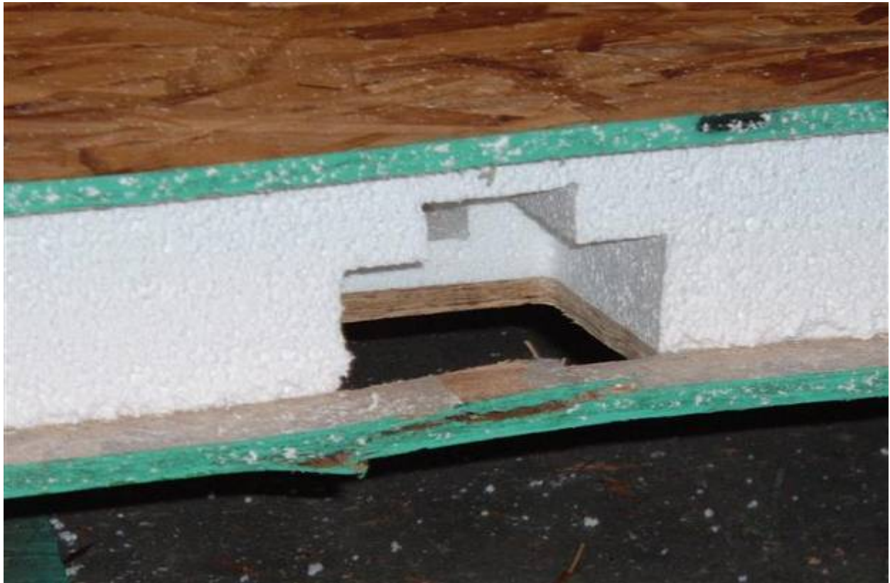
FIGURE C2. AXIAL LOAD (COMPRESSION) TEST (Initial buckling failure on compression side through electrical chase holes - typical)
