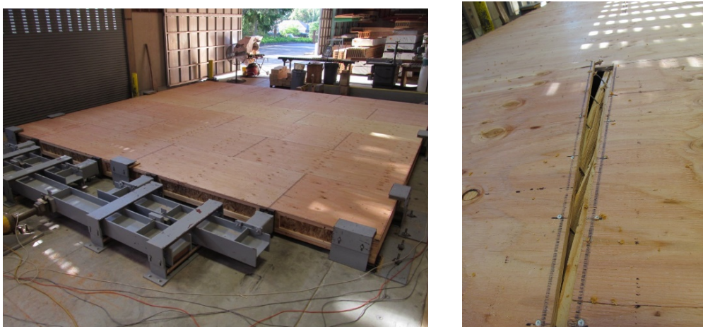
Figure 7. Diaphragm failure modes (Case 1 Unblocked)
