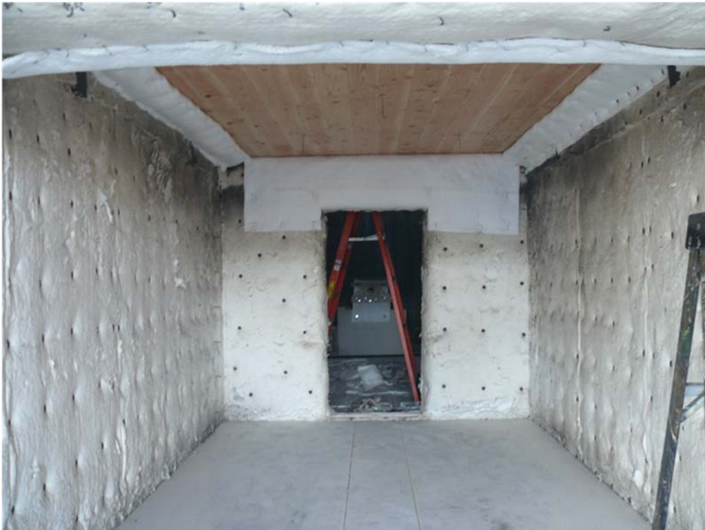
Figure X2-6. Picture Illustrating Ceramic Fiber Cover around Panel Perimeter
