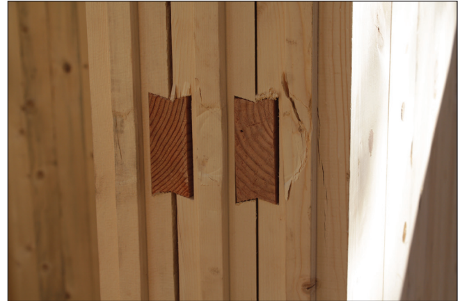
ICLT panel optimization to three-layer assembly.
