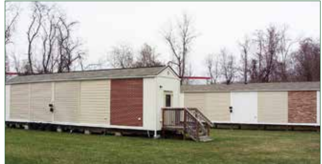
Figure 1—Test buildings No. 1 (right) and No. 2 (left).
