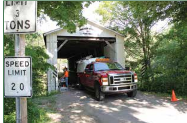
Live-load testing on a covered bridge.
