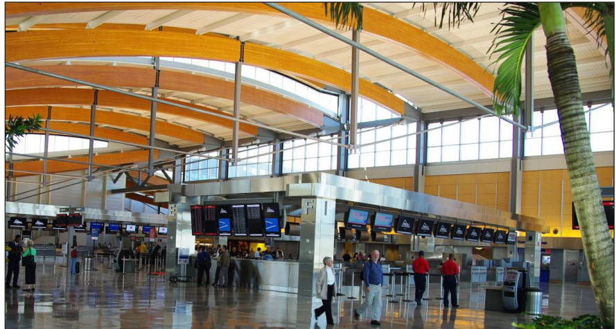
A wood roof structure for Raleigh–Durham Airport Terminal 2 resulted from the use of the Athena Impact Estimator for Buildings LCA software tool in determining which design option had the least environmental footprint. Photo: Arup.
