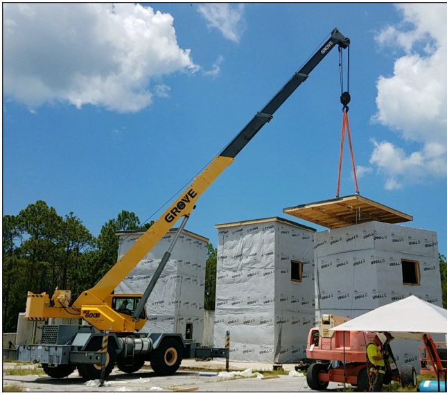
Temporary moisture protection added to CLT blast testing structures.
