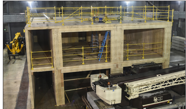
Figure 1. Superstructure of the CLT building in the ATF laboratory.
