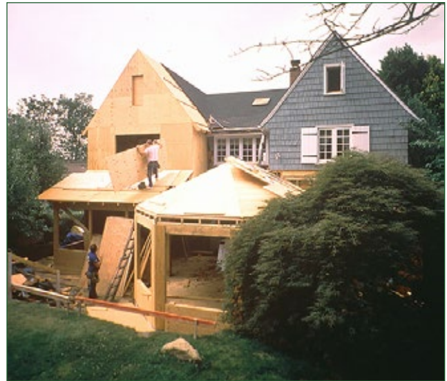
Repair and remodeling of an existing residential home.
