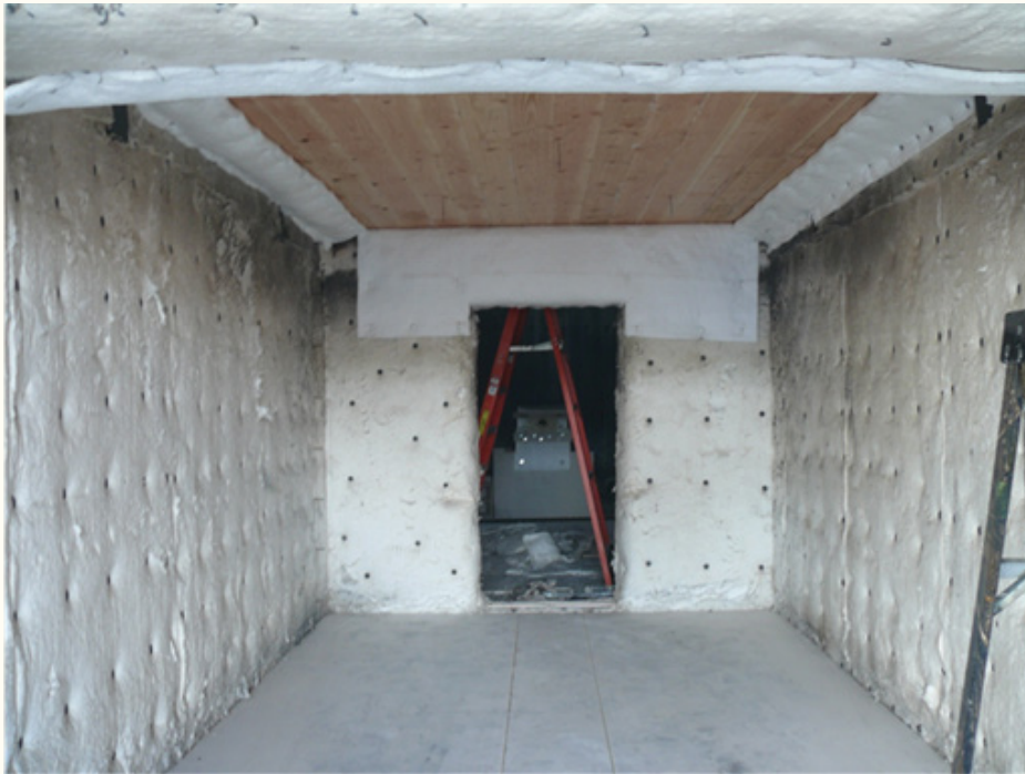
PICTURE ILLUSTRATING CERAMIC FIBER COVER AROUND PANEL PERIMETER
