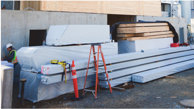
Figure 24 Material Handling and Storage.
