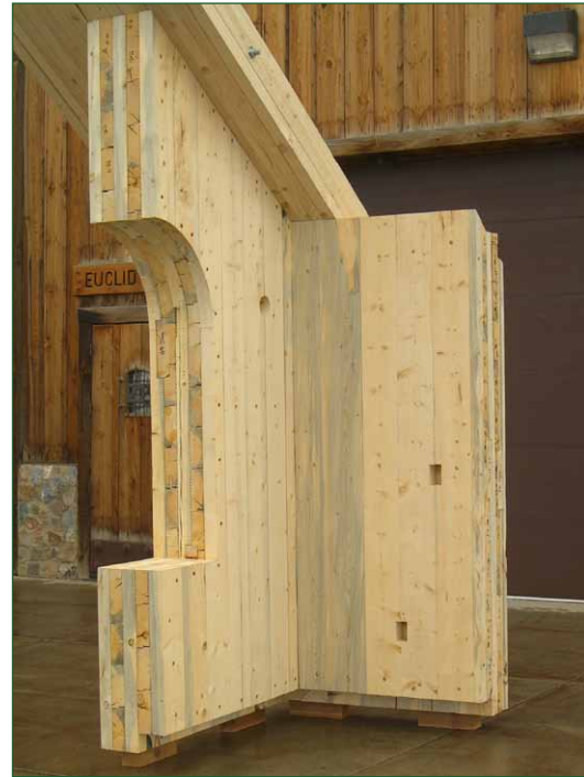
Figure 1. Prototype of a mechanically fastened CLT wall section made from beetle-killed wood.
