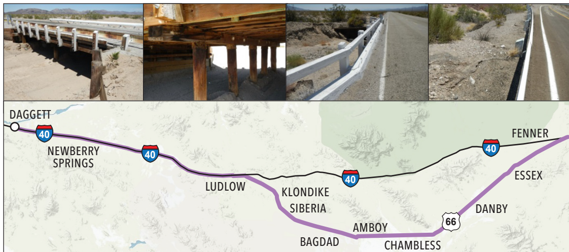
Original design features of the timber bridges located along historic California Route 66 (highlighted in purple) include standard 19-ft simple spans, timber pile/cap intermediate supports, timber bridge railing and curb system, and a flexible metal approach railing mounted on timber posts.
